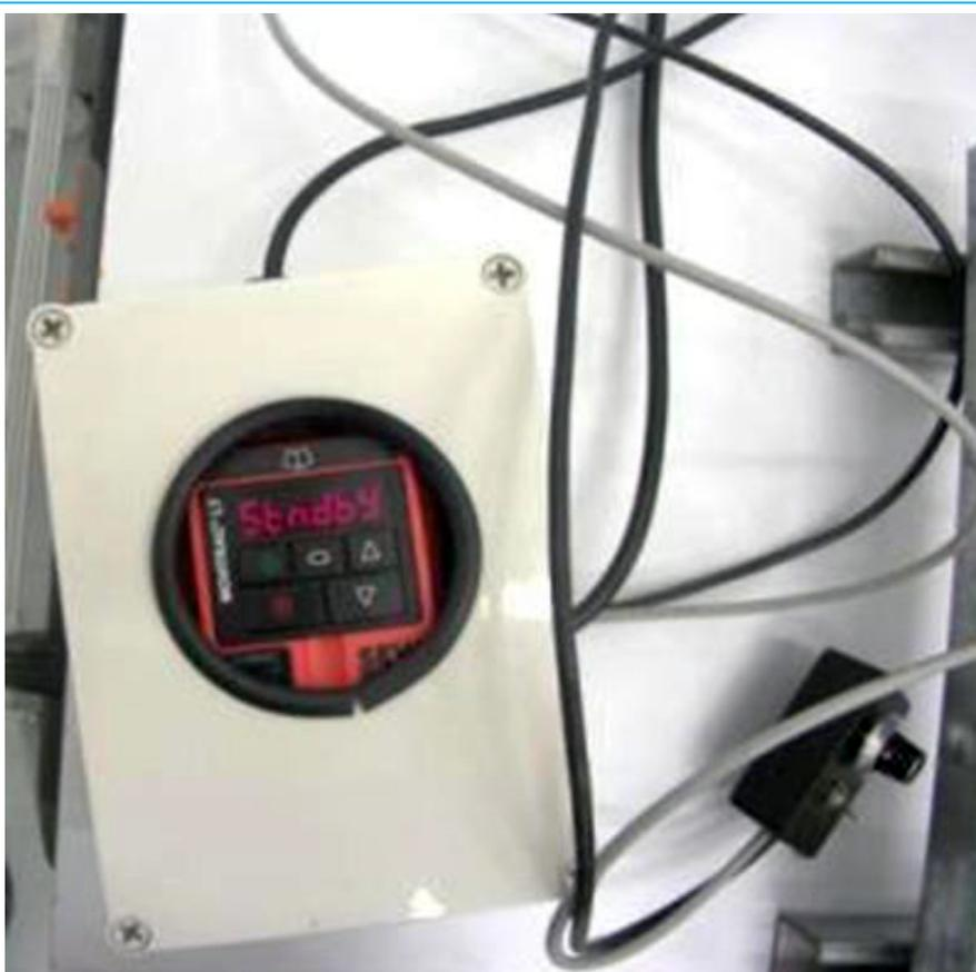
Fig. 5 The VSD, cable and potentiometer with rotary dial and on/off switch.
